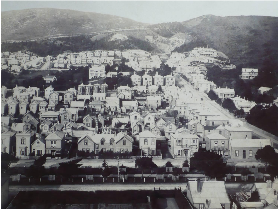
The former Gray Estate can be seen, still uninhabited, on the left just above the middle of this photograph dated c. 1895. Poutawera's house would be just out of the frame to the left of the 'green' patch. (Note Waring Taylor's large house far right.) [Photograph from the collection of Alan Marshall]
