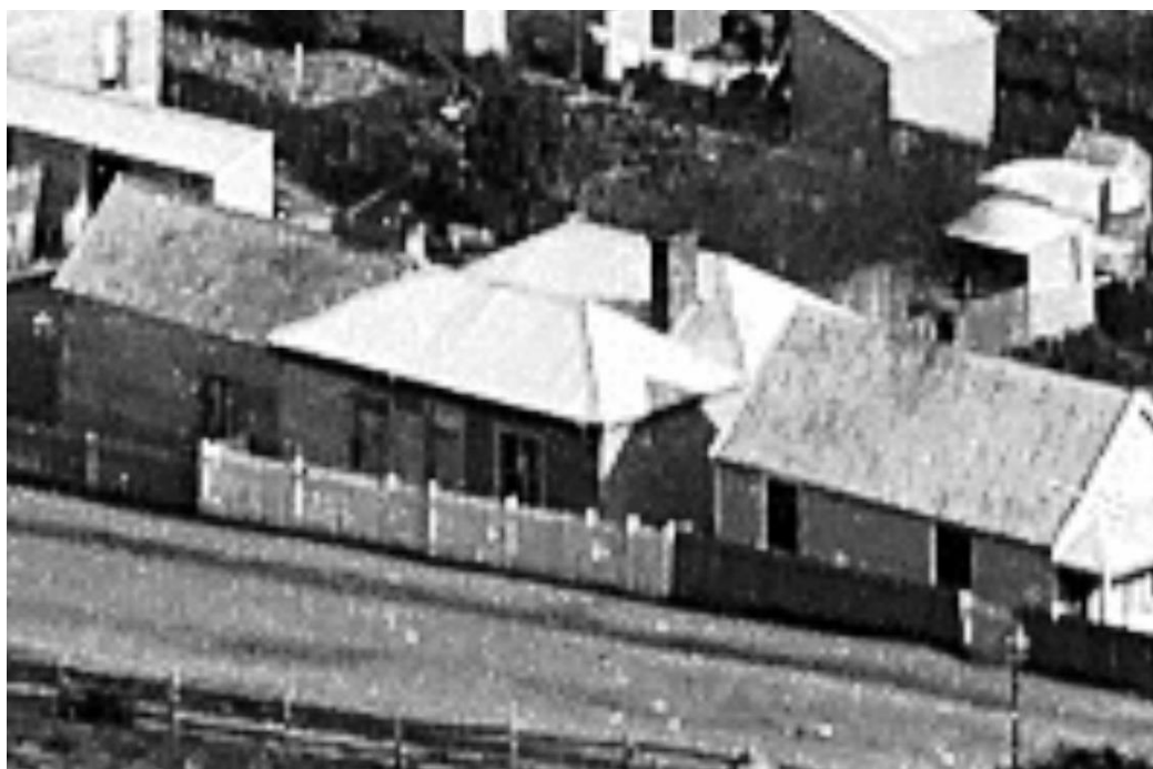
The original corrugated iron roof of no.38 is a contrast with the shingle roofs on the houses either side in this detail from an image taken in 1884. The other two houses no longer exist. (BB-2235-1-1-G, Alexander Turnbull Library)
