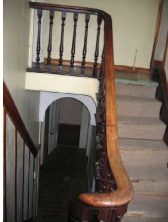
Servant's stairs, J Newman, 2008.
