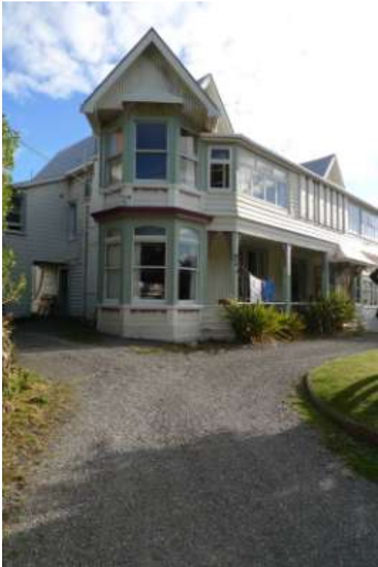
Main entrance, north west elevation, R Murray, 2010.
