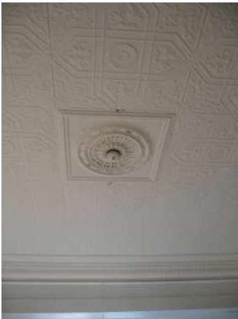
Pressed tin ceiling, Archbishop's room, J Newman, 2008.
