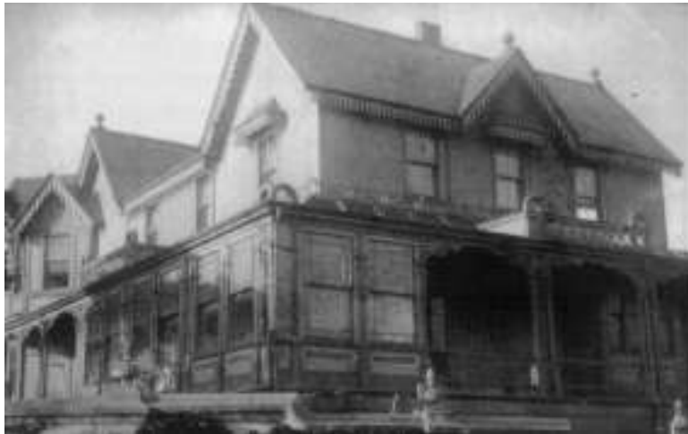
"The verandahs have been given a juicy assortment of decoration including brackets, lattice work, pierced balustrading and bold expanses of glazing" (Terence Hodgson, Proud Possessions )
